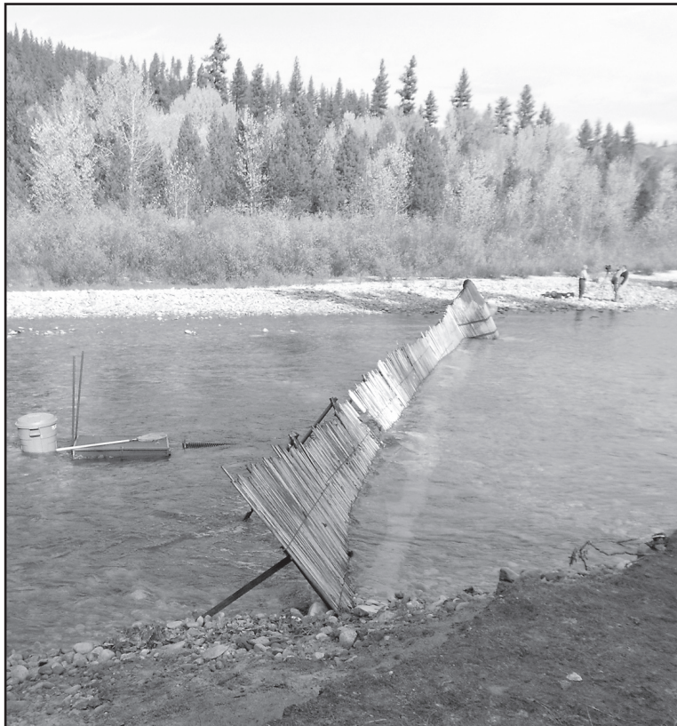
The weir stretched across the North Fork of the Boise River and detains spawning fish in trap boxes. Photo by Eileen Capson.
